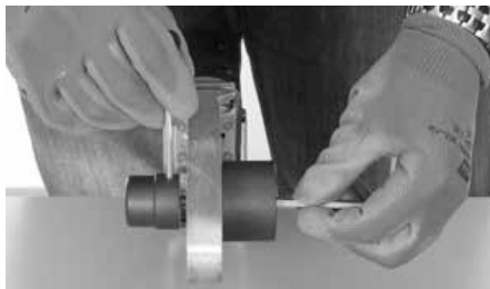
1. Persiapan Welding Machine
